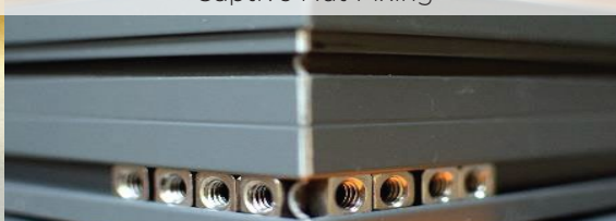
Captive Nut Fixing
